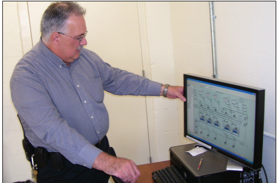
General Services Division Maintenance and Operations Manager Dave Parsons demonstrates the real-time monitoring of units at the chiller plant. The General Services Division has begun real-time remote monitoring of heating and cooling of more state buildings.
