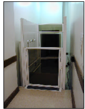
Pictured is the new ADA lift in the east wing across from the State Treasurer's Office.
