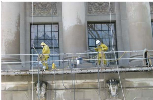
Work crews keep busy around the Capitol's main building as they are in the midst of a major cleaning and restoration process of the building's exterior, using special techniques and treatments to restore the Indiana limestone.
