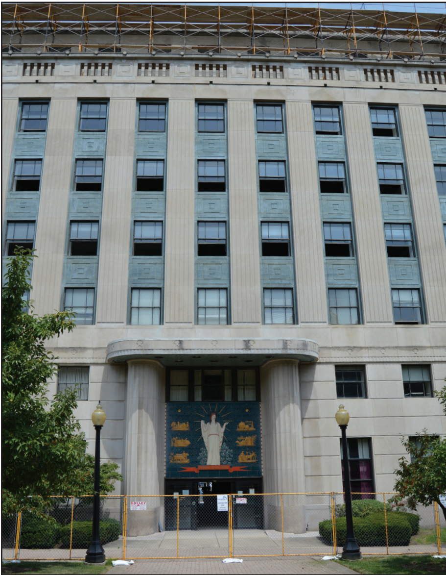
Renovations began in July on Building 3, popularly known as the DMV Building.
