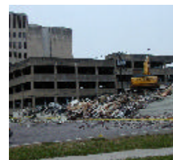
Parking Building Demolition
