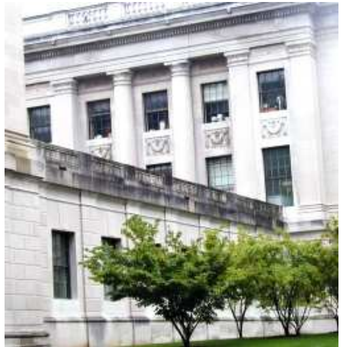
[ABOVE] Dirt and grime on parts of the Capitol Building are obvious signs that the exterior must be cleaned. However, other signs that are not as obvious are the cracks in the joints.
